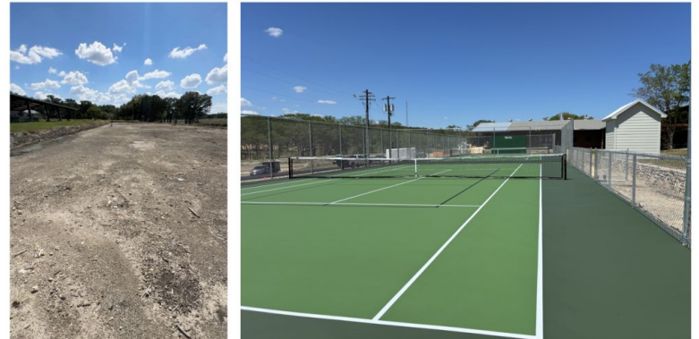
CAMP LA JUNTA BEFORE AND AFTER
